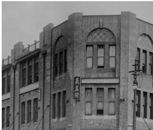
D - EXISTING BRICKWORK 96-100 HAY STREET
