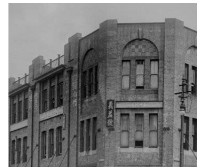
D - EXISTING BRICKWORK 96-100 HAY STREET
