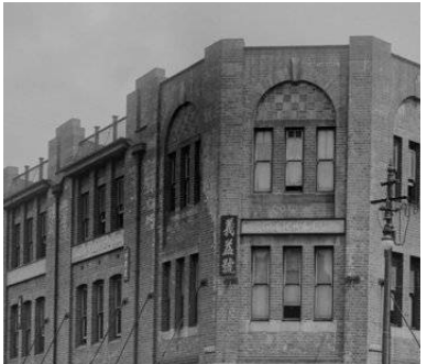
D - EXISTING BRICKWORK 96-100 HAY STREET
