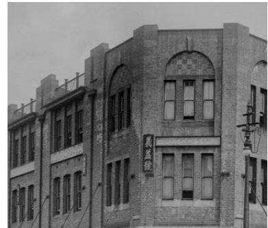
D - EXISTING BRICKWORK 96-100 HAY STREET
