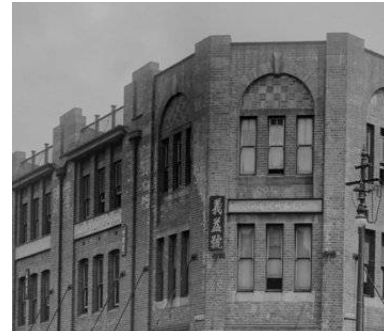
D - EXISTING BRICKWORK 96-100 HAY STREET
