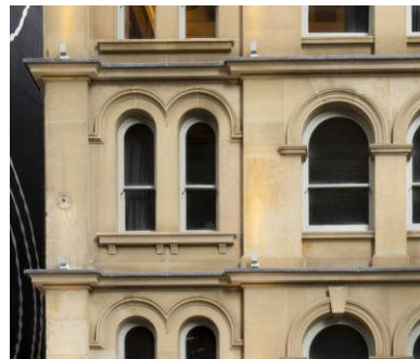
E - TIMBER DOUBLE HUNG WINDOWS PORTER HOUSE - CANDALEPAS ASSOCIATES
