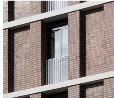
A - DRY PRESSED BRICK REGENT STREET - CANDALEPAS ASSOCIATES
